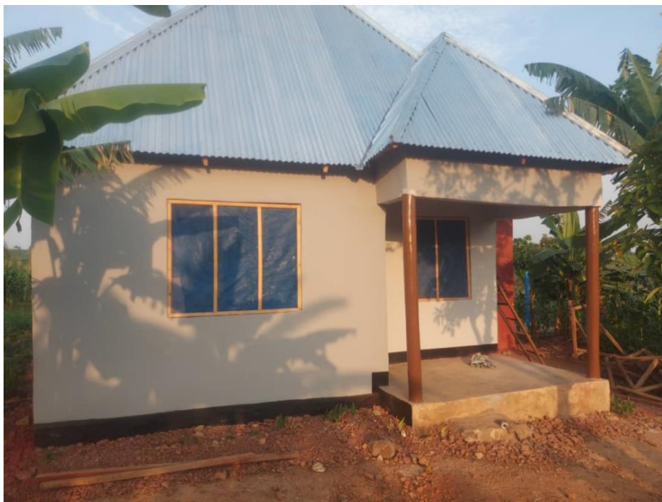
Figure 3 The view of the house after completing the construction
